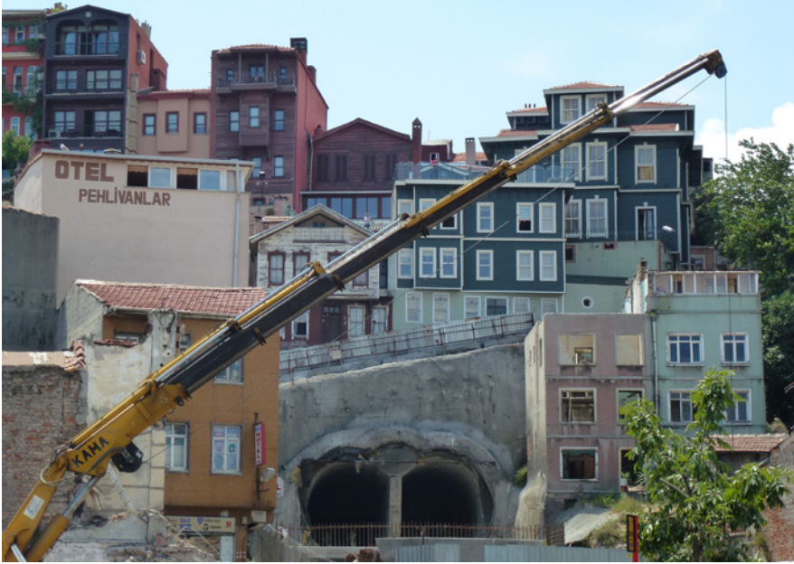
Metro construction in a World Heritage district in Istanbul. (Photo: V. Marquart, 2012)
