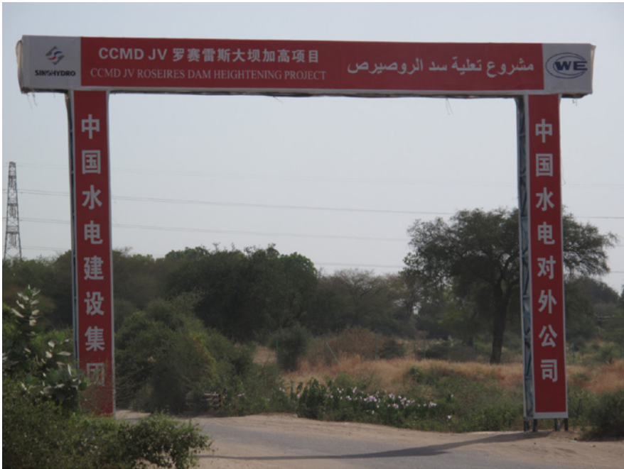
As one approaches the Roseiris Dam Heightening Project by road, this gate makes it unmistakably clear that the company charged with it is Chinese. (Photo: G. Schlee, 2009)
